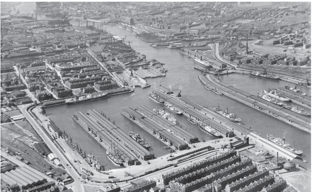
Prince's Dock, the largest on the River Clyde when it opened in the 1890s, and the embarkation point for the Bains who emigrated to Canada. It had three basins – South, Centre, and North – that lay parallel to the Clyde, and a Canting Basin connecting them, which provided access to and from the river. The ships of the Allan Line generally sailed from the North Basin, the right-hand basin in the photograph. The dock was located in the Govan area of Glasgow on the south bank of the Clyde, which runs east-west through the photograph to the Atlantic Ocean. Residential tenement housing can be seen in the foreground. The Queen's Dock can be seen on the north bank of the Clyde on the middle-right-hand side of the photograph, which was taken on 4 July 1936 and is in the Historic Environment Scotland Aerofilms Collection. See p. 71, n. 55.
